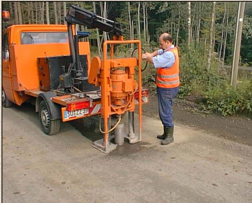
Core drilling
